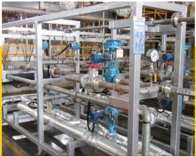
Adjustable oxygen flow control skid
